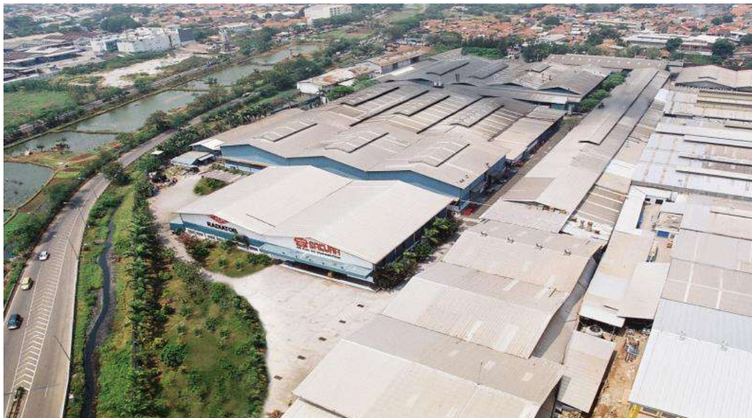
Kapuk Plant (Radiator Facilities)
